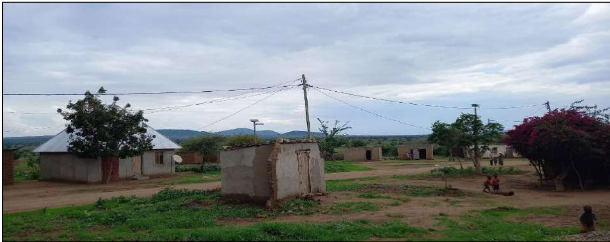
Figure 7: Part of the Mini-grid Distribution Network at Ngutoto Village
