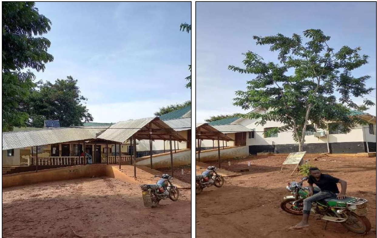
Figure 10: Kibindu Public Health Centre Powered by Solar PV-Gasifier Hybrid Mini-grid
