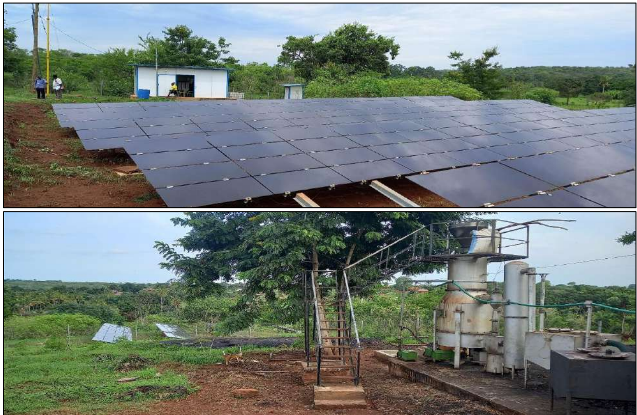
Figure 9: Solar PV -Gasifier Hybrid Mini-grid at Kibindu Village
