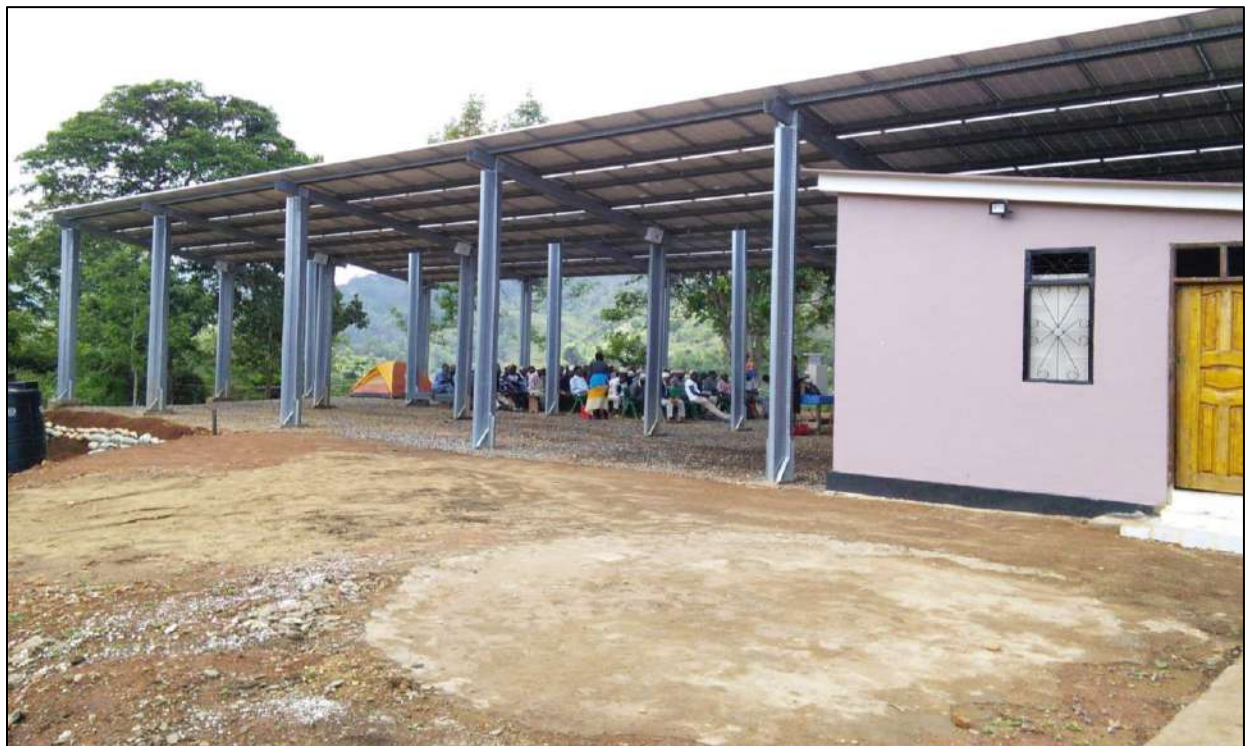
Figure 15: Customers Meetings under the roof of 48kW Mpale Solar PV Mini-grid Customer Aspects
