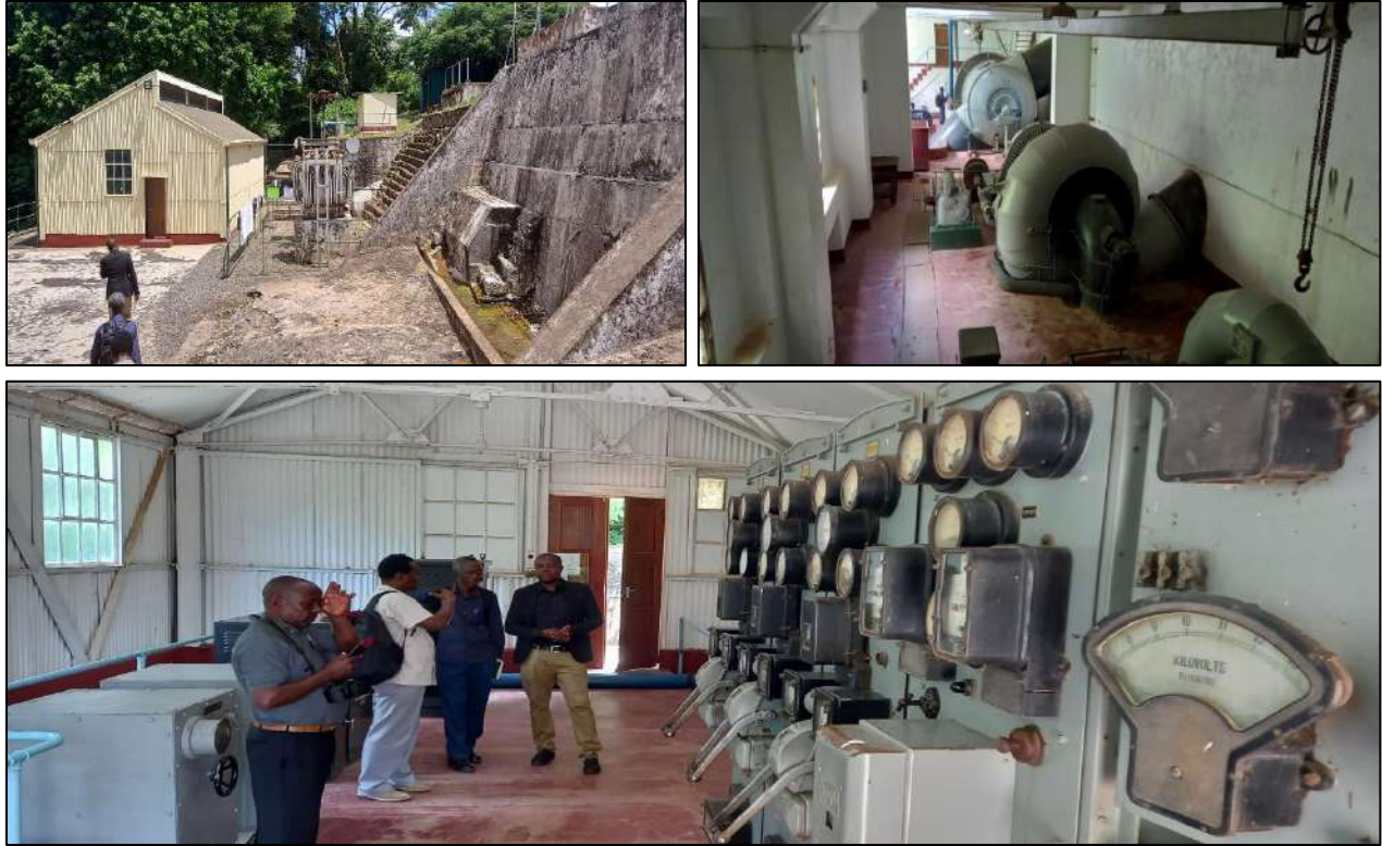
Figure 12: Obsolete Kikuletwa Hydro Power Plant in Kilimanjaro Region
