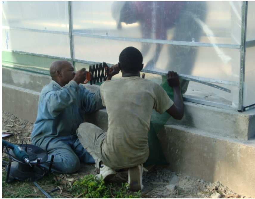
Figure 6: Technicians fixing the air inlet vent of green wire mesh
