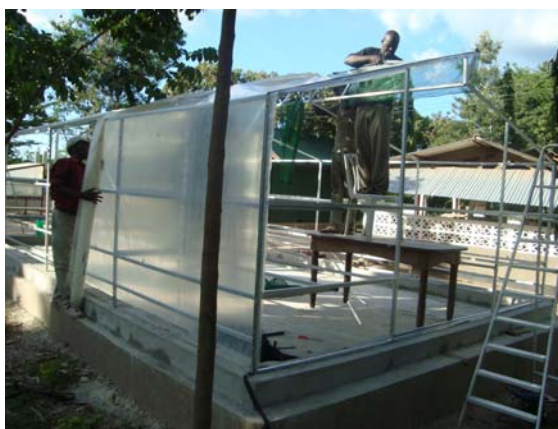
Figure 4:Technicians fixing visqueen sheet on the structure of solar dryer
