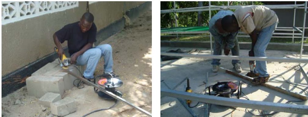
Figure 1: Activities for construction of Semi Industrial Solar Dryer (SISD)
