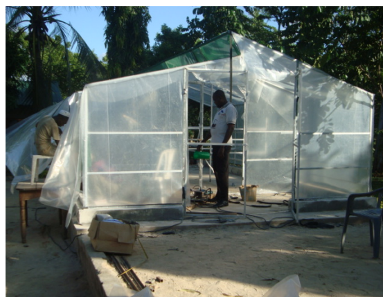
Figure 4:Technicians fixing visqueen sheet on the structure of solar dryer
